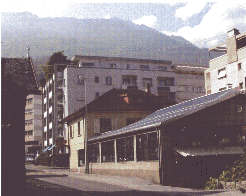
The Stained Glass Arts College is located in an industrial building in Monthey, surrounded by the Alps, seen in the background.
